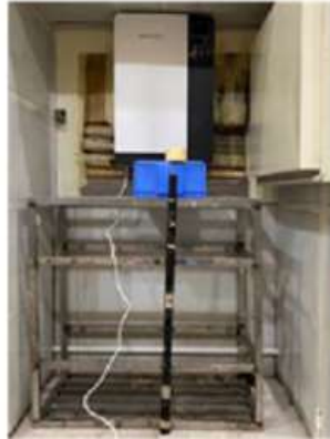
1.5M below ventilator
