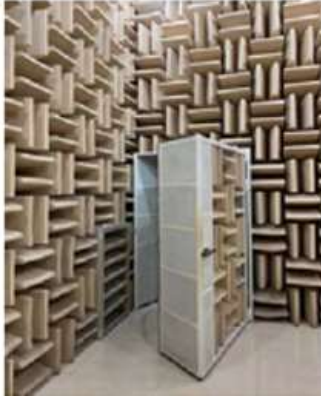
Semi anechoic room
